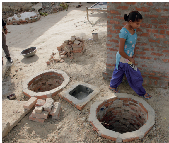
Twin-pit toilet constructed in Gonda, Uttar Pradesh
